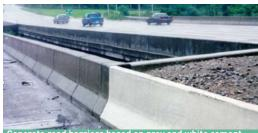
Concrete road barriers based on grey and white cement, respectively, illustrating the visibility advantage of white concrete under wet conditions.
