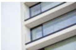
Exterior facade panels and decorative coating stones, Belgium
