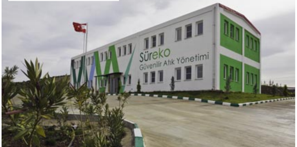
Waste treatment plant in Kula, Türkiye
