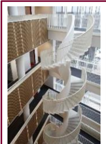
5. UHPC staircase in Per Aarsleff office building, Denmark
