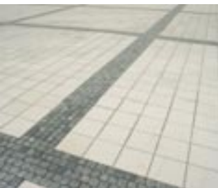
Floor tiles, white cement, Norway
