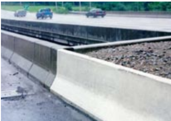
Fig. 8: Grey concrete road barriers painted white. This illustrates the safety hazard and additional costs needed for repainting the road barriers.
