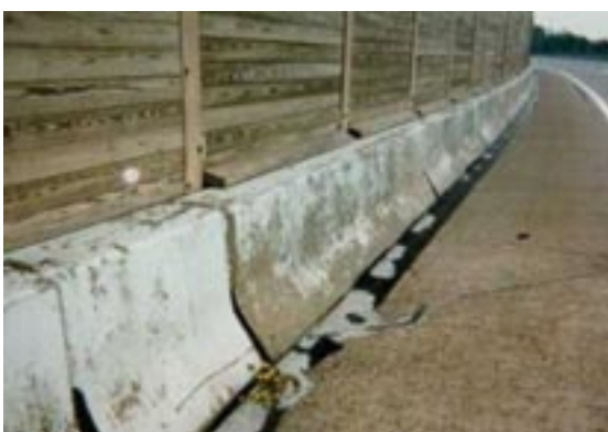
Fig. 8: Grey concrete road barriers painted white. This illustrates the safety hazard and additional costs needed for repainting the road barriers.
