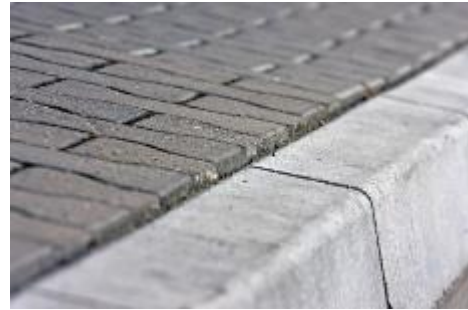
2. Paving blocks: Kerb, Poland
