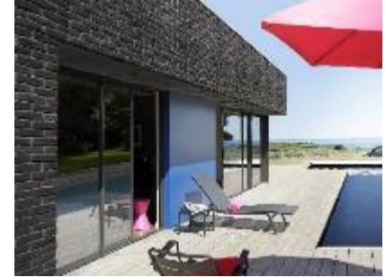
3. Artificial stone: Villa façade application, France
