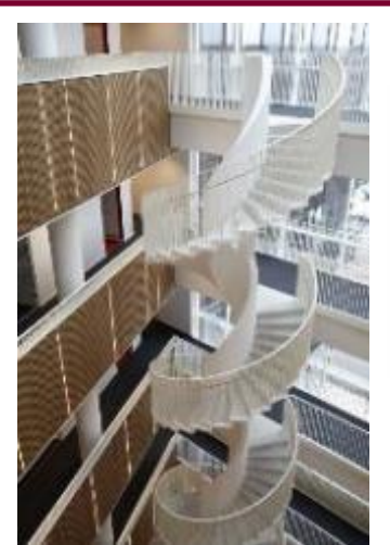
5. UHPC staircase in Per Aarsleff office building, Denmark
