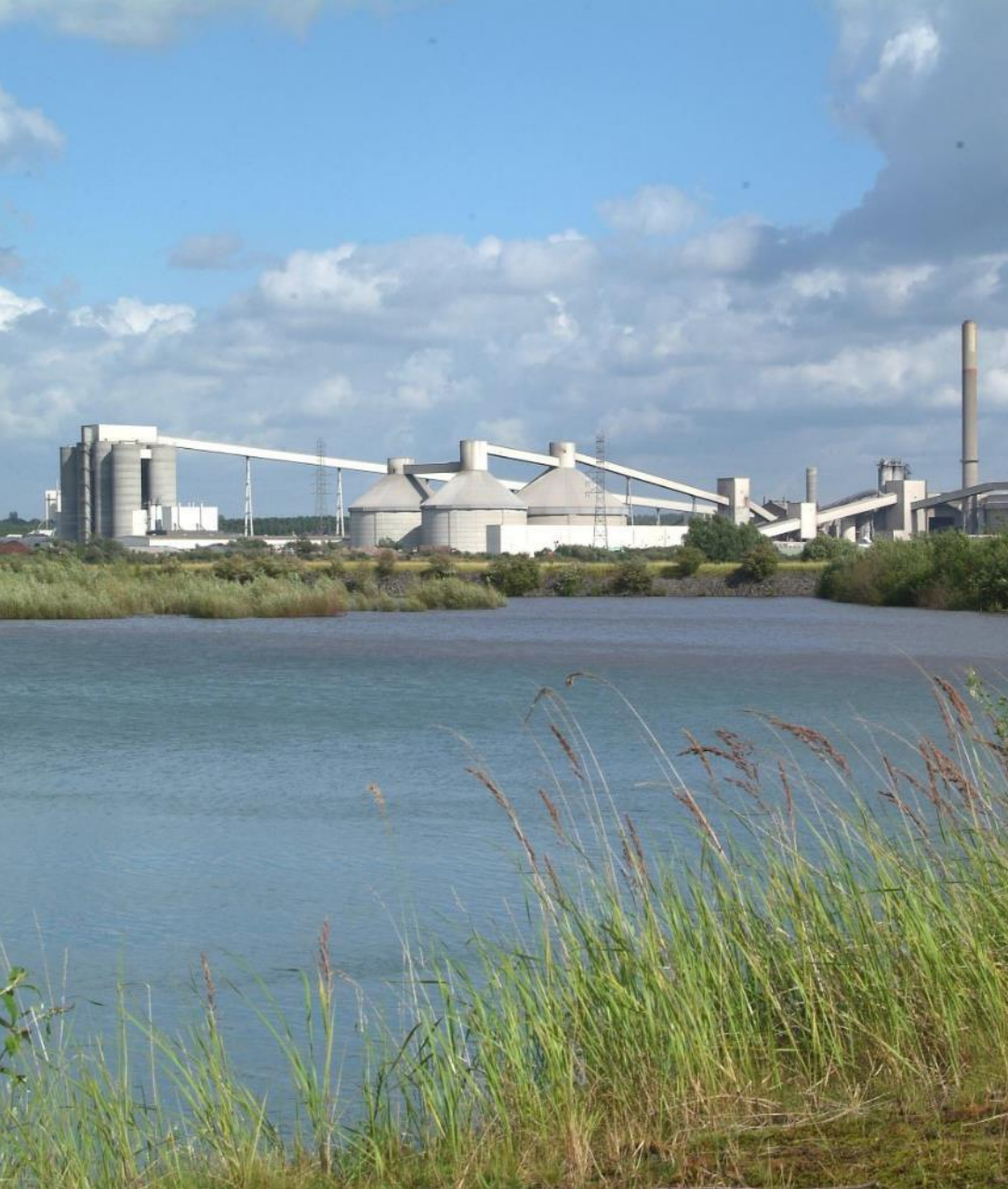
Gaurain Plant, Belgium
