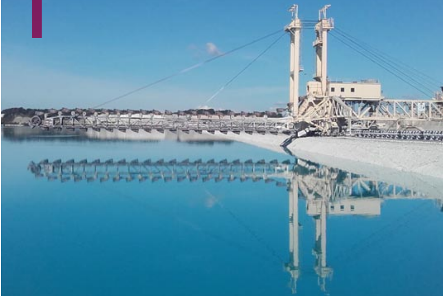
Dredger at Aalborg plant, Denmark
