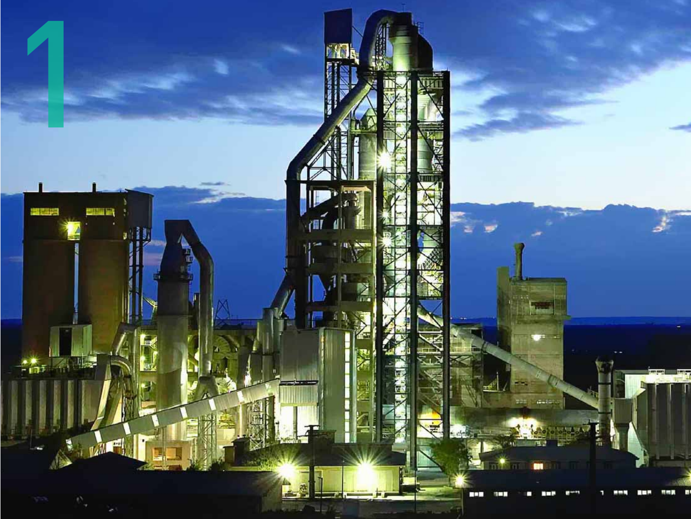
Cement plant in Edirne, Turkey
