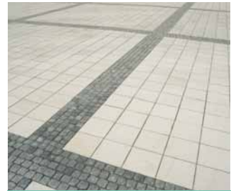
Floor tiles, white cement, Norway
