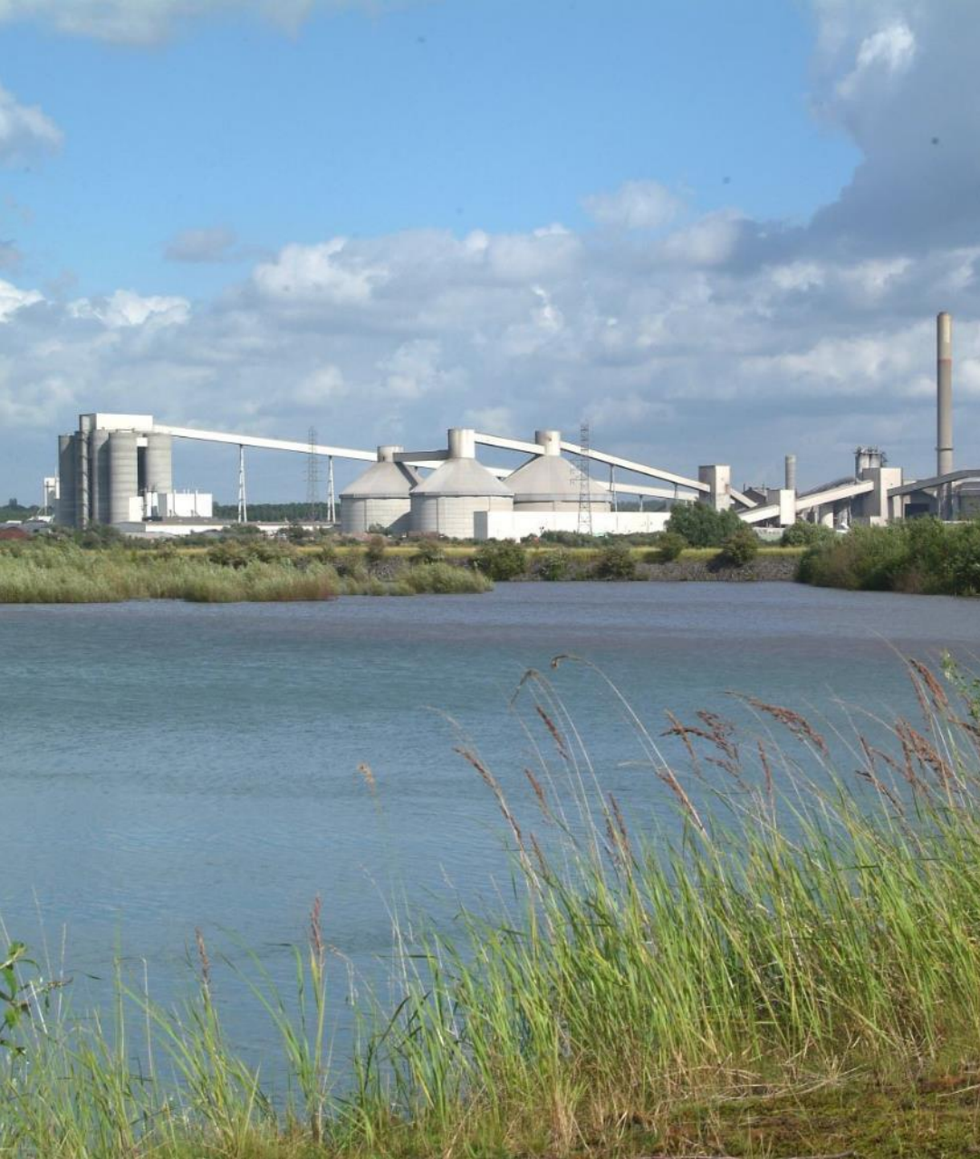
Gaurain plant, Belgium
