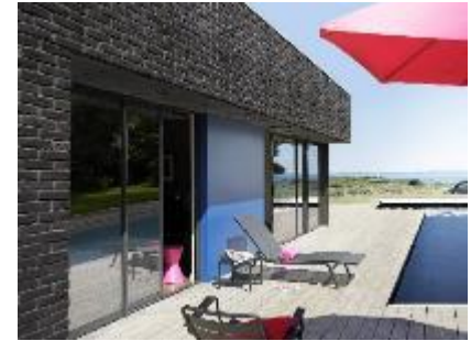
3. Artificial stone: Villa façade application, France
